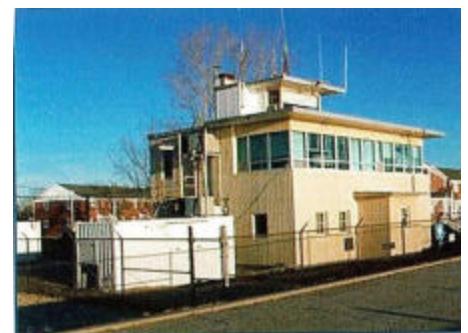
Combatant Craft Division Waterfront Operations Facility, Ft Monroe. U.S. Navy Photo.
