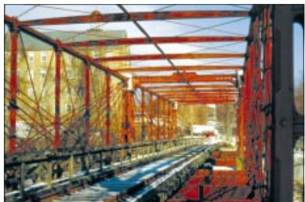
Bollman Truss Bridge — designed around 1870 by Wendell Bollman, "master of the road." Many of this type were built, but this is the only survivor and is now used only for pedestrians; located at Savage Mill, MD, on a branch of the Washington Line.
