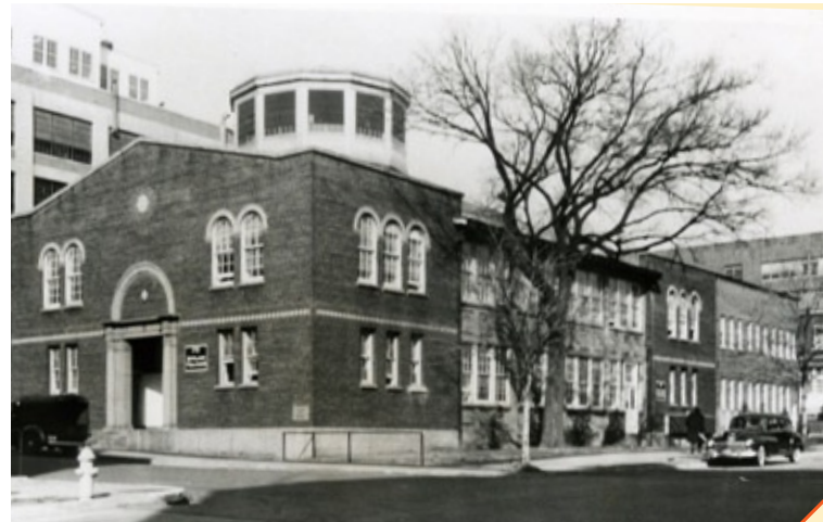
Navy Mine Unit Building, Washington DC Naval Yard
